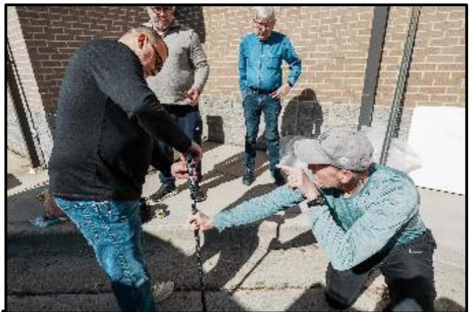
SK Villareal and Tim Albers assemble gas pipe for fryers
