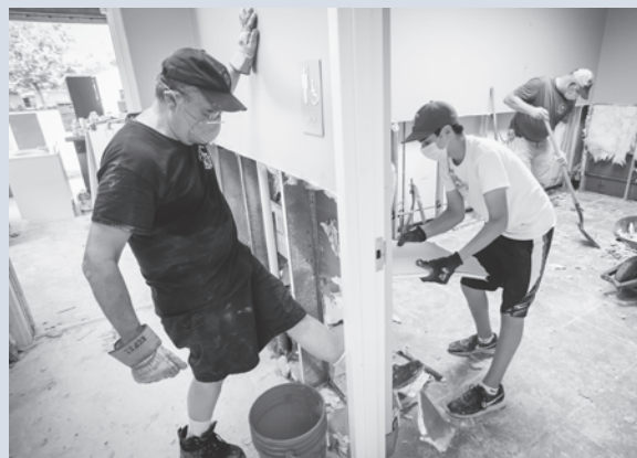
Knights from Our Lady of the Lake Council 9240 in Mandeville, La., remove water-damaged wallboard and flooring in one of their parish's rooms as part of a cleanup effort.
