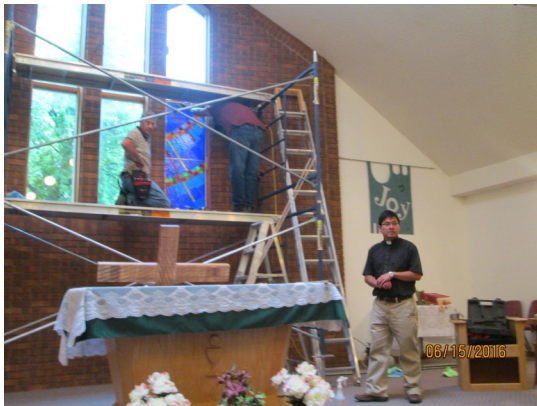
First Pane of glass replaced.
