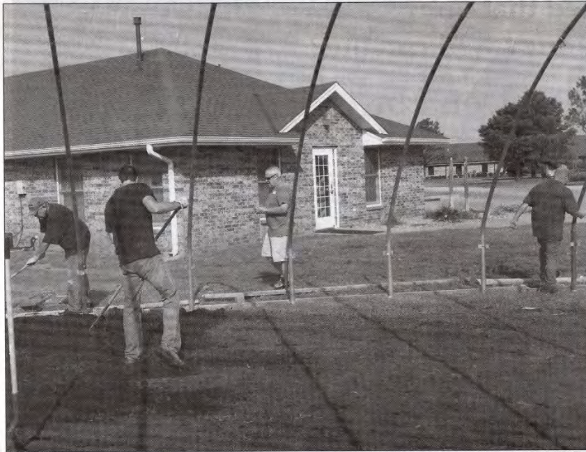
Since our last issue, the Knights from Council 11237 ( Edmond, St. Monica ) helped with the construction of a new greenhouse at the Center of Family Love. The CoFL residents will be using this greenhouse for their winter crops.
