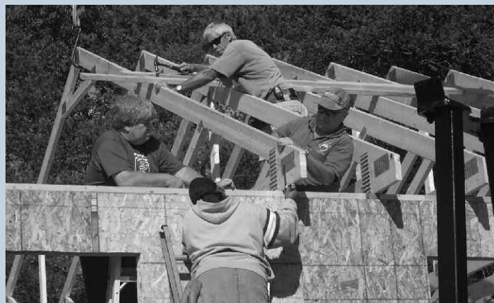
Members of St. Joan of Arc Council 12054 in Ridgely, Md., install supports for the roof of a house built through a local Habitat for Humanity project.
