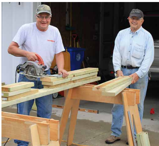
Joe Elbert (left) and Ron Wolf begin the large task of cutting the lumber for the wheelchair ramp.
