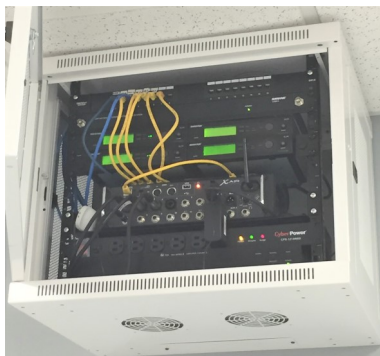
System Component Cabinet
